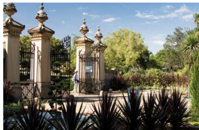
The Woolloomooloo gates today
